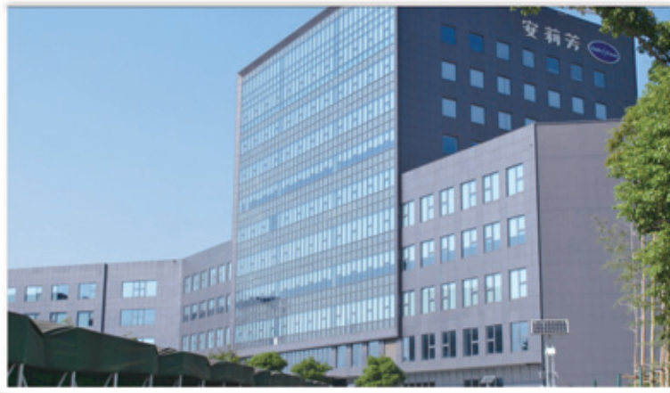
Windows and glass curtain walls are made of insulating broken bridge glass, reduce the loss of cool air.
